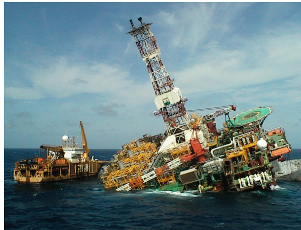
Figure 2.4.: The Petrobras P-36 oil platform sinking.
